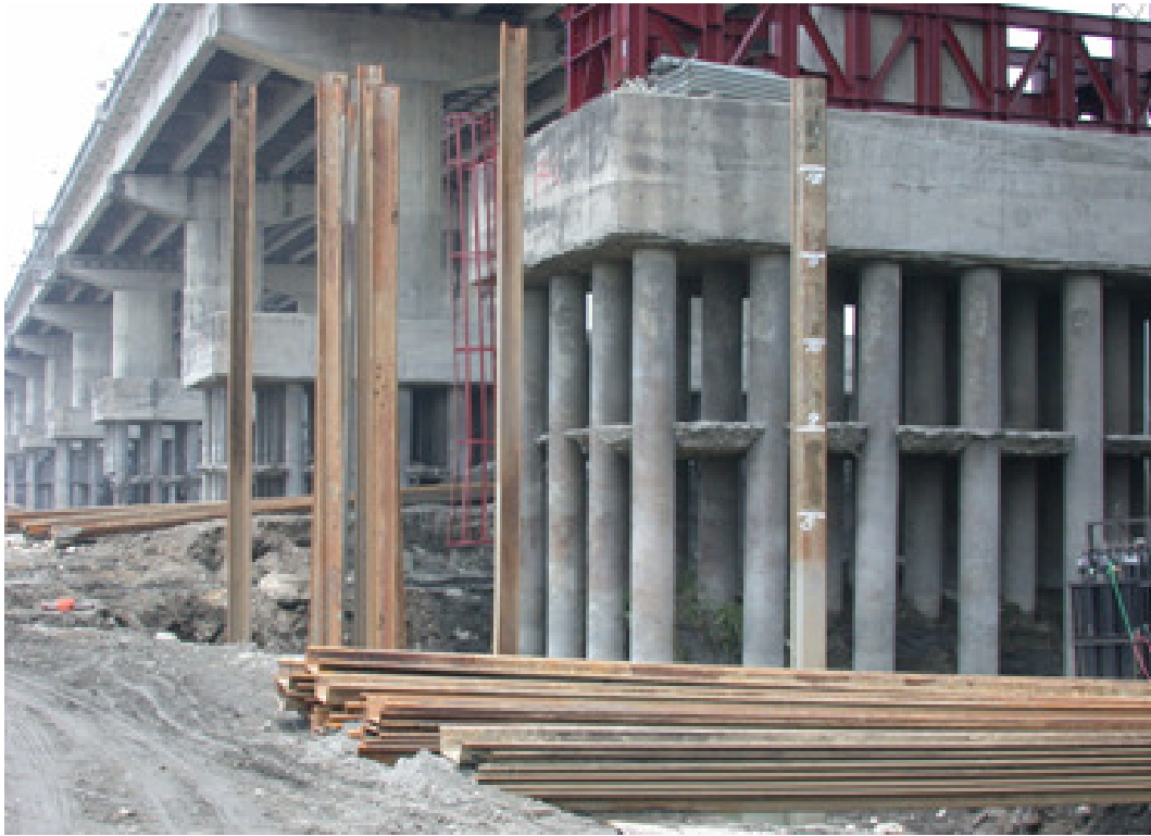
Figure 6. A bridge on a low shear strength soil riverbed that remained stable after group pile foundations were severely exposed (Sijhou Bridge, Changhua, Taiwan).
