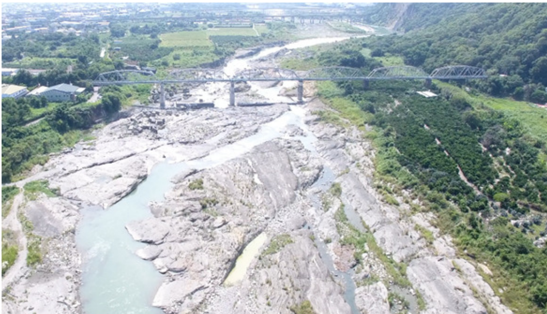
Figure 1. A bridge across a high shear strength rock riverbed with shear bandings.
