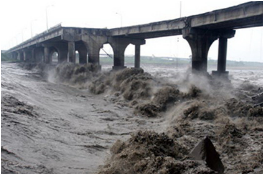
Figure 4. The collapse of Houfeng Bridge in Taichung, Taiwan, during Typhoon Sinlaku in 2008 (Jeng, 2008).
