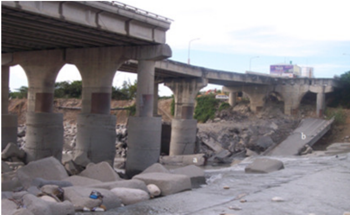
Note: In the figure above, a is the toppled caisson, and b is the fallen bridge deck.
