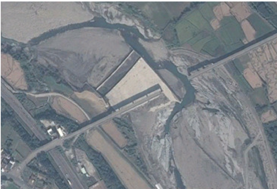
Figure 13. Satellite image of the partial drop of the Zhongzheng Bridge in 2013 (Google Earth, 2020).
