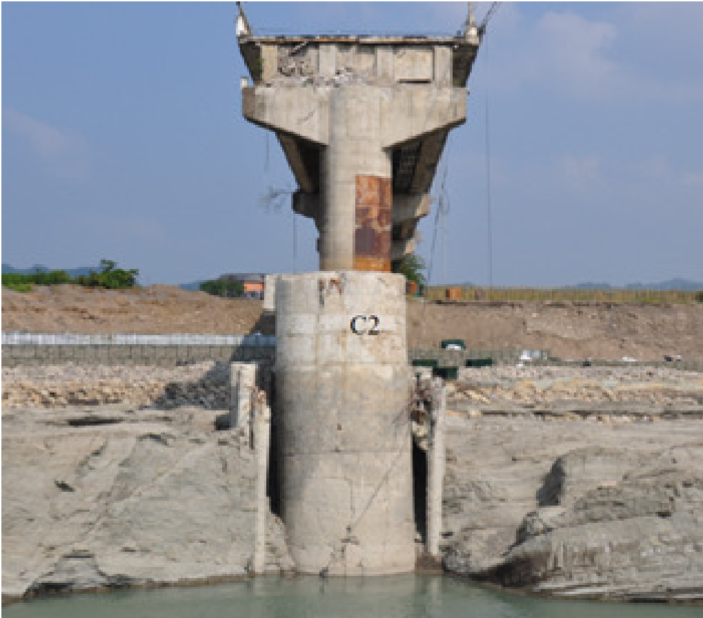
(c) Stepped deep grooving of shear-band rock riverbed after Typhoon Soulik in 2013
