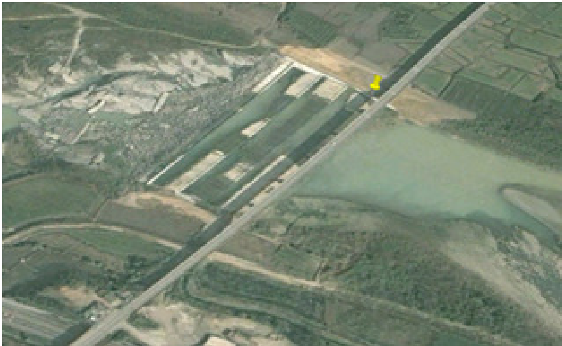
Figure 11. The construction of a concrete-groundsill downstream of the Zhongzheng Bridge completed in 2003 (Google Earth, 2020).
