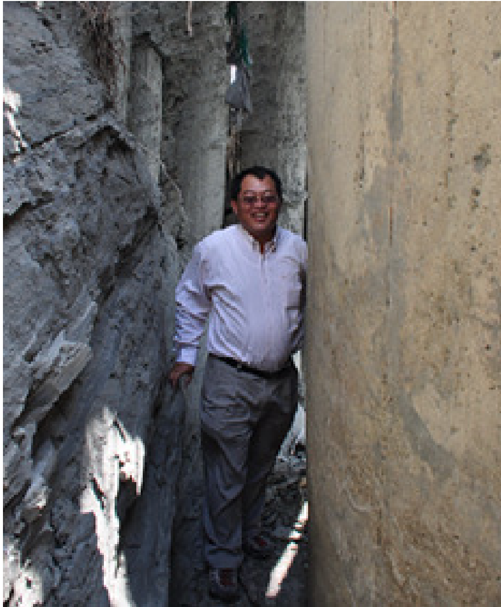
(d) The annular empty space that appeared after the loss of shear-band rocks that bounded the C2 caisson in Figure 23(b)
