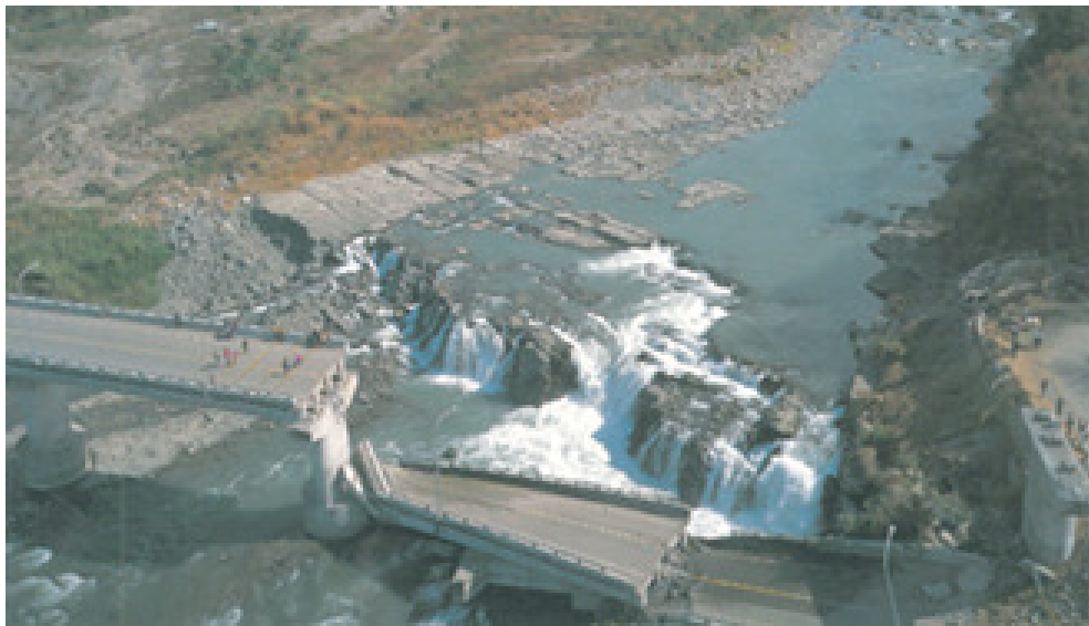
Figure 3. The collapse of Pifeng Bridge in Taichung, Taiwan, during the 1999 Jiji earthquake.
